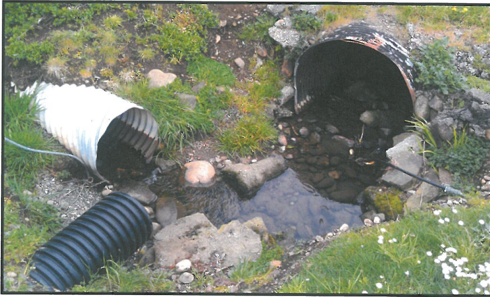
Figure 1.4.2: 48-inch CMP Culvert Inlet Structure
