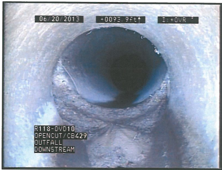
Figure 1.4.4: Separated Joint in Outfall at 429 Buena Vista Loop
