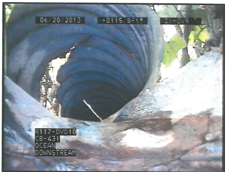
Figure 1.4.4: Separated/Broken Joint in Outfall at 431 Buena Vista Loop
