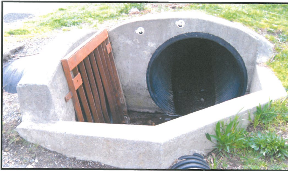
Figure 1.4.1: 48-inch HDPE Culvert Inlet Structure
