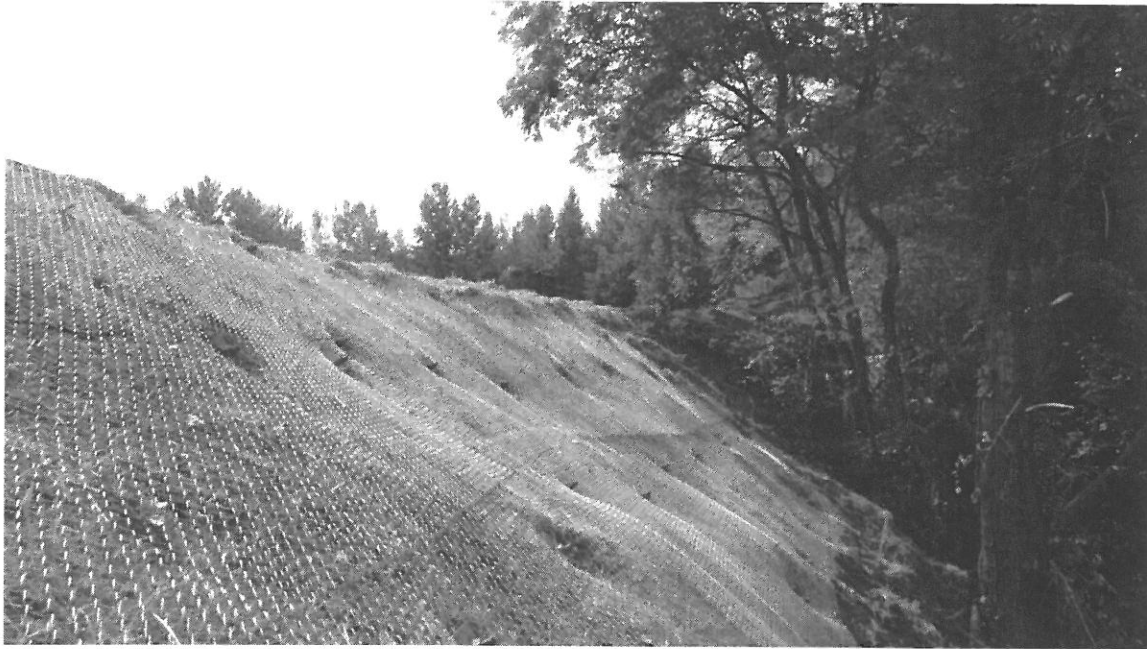
Photo of Soil Nail and High Strength Mesh Facing Reinforcement
