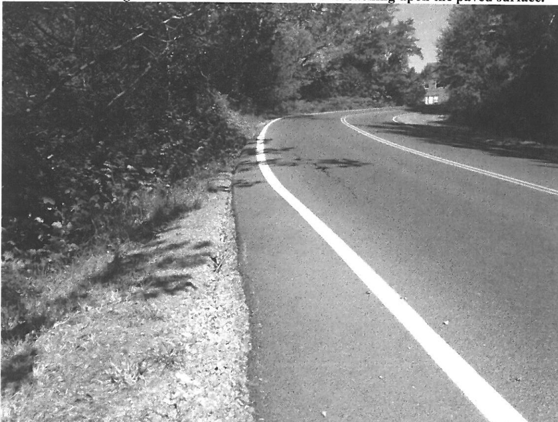
Photo illustrating the outboard shoulder failure encroaching upon the paved surface.
