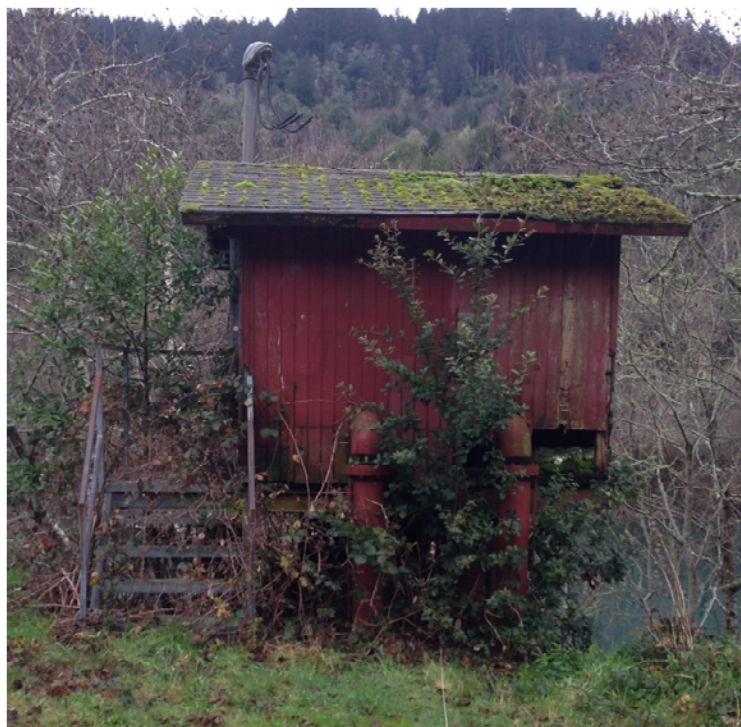
Figure 3.3.1 – Abandoned intake station on the Chetco River (Tide Rock Intake Station).
