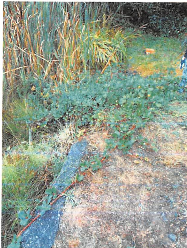
Partially buried spillway control section
