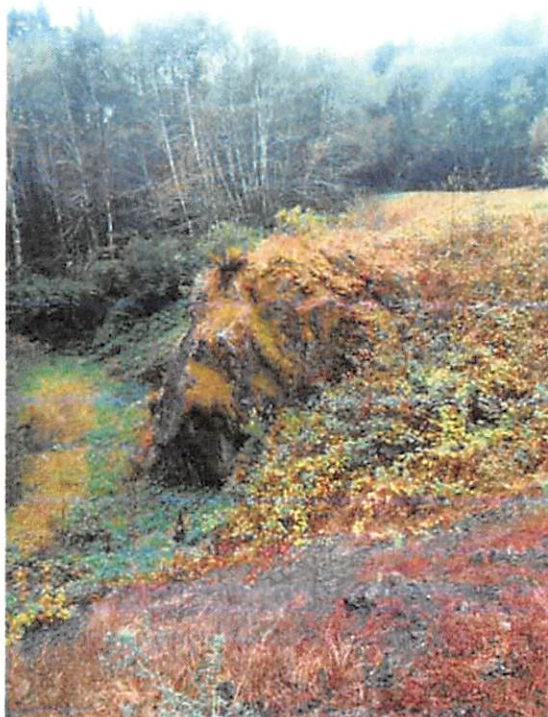
Vegetation on the downstream slope, right abutment and toe of the dam
