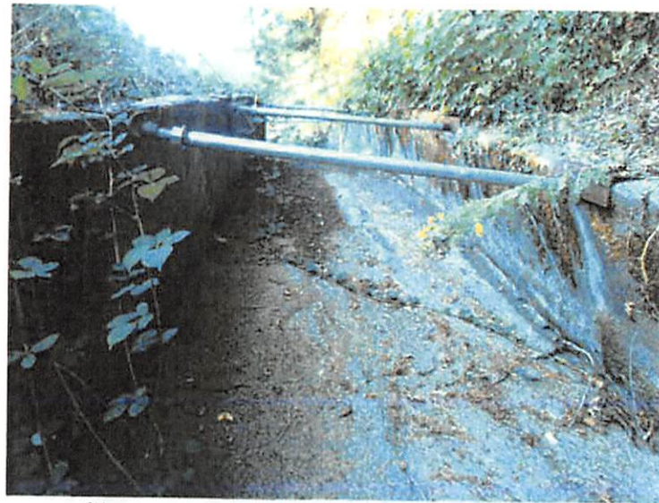
Slope movement into spillway control section
