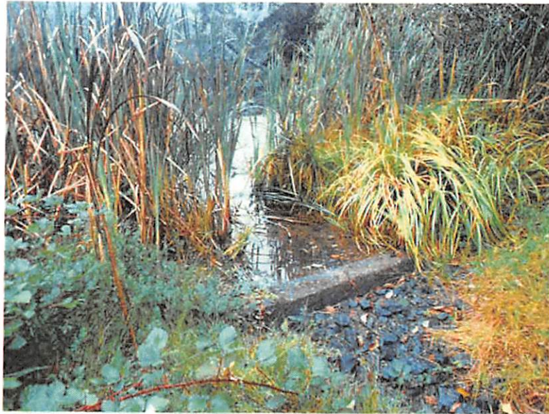
Vegetation in the emergency spillway control section
