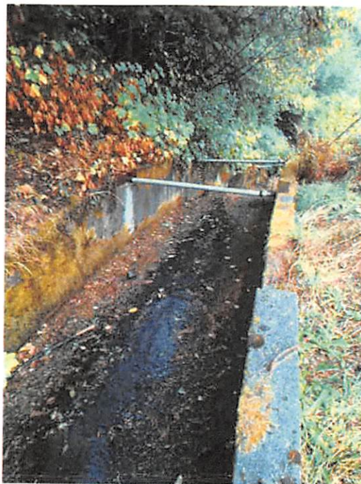
Steel struts preventing spillway channel retaining wall failure
