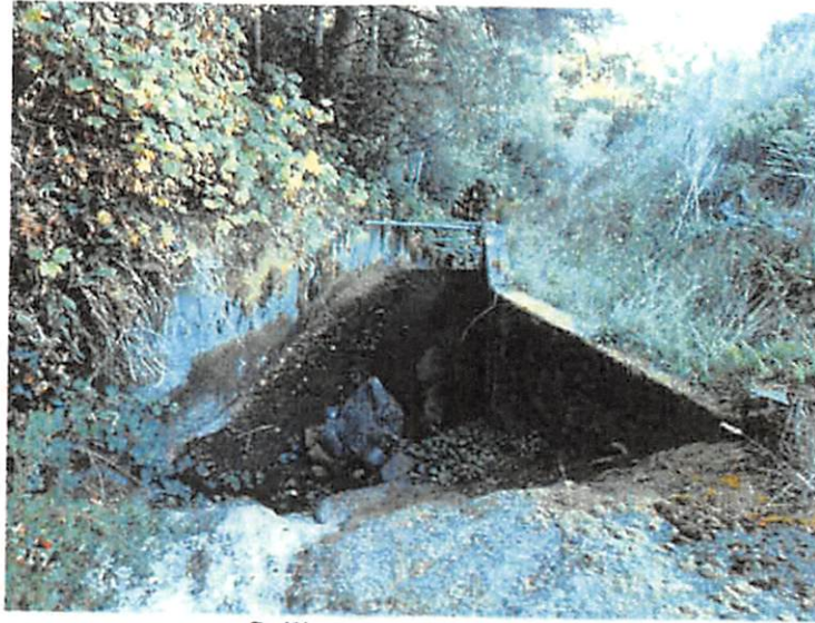
Spillway control section
